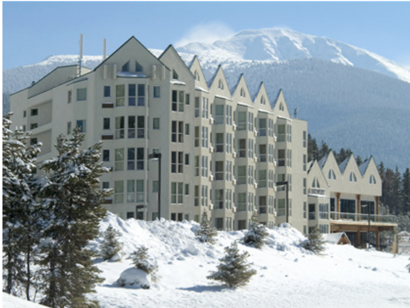
A renovation and facelift tripled the size of this hotel and resulted in a new entrance, landscaping and parking facilities.
