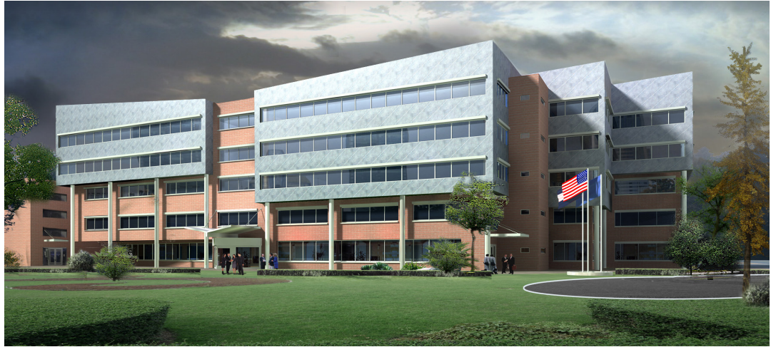
Sustainable elements such as reduced parking footprint, increased open space and extensive daylighting restore health to the medical facility.
